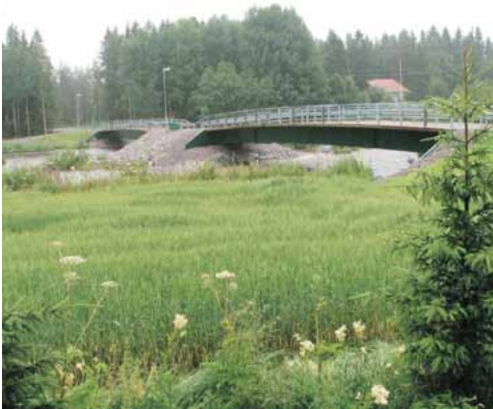
Hollanti private road bridge
